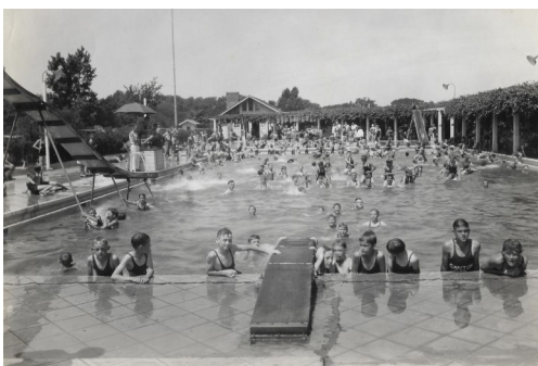
Old Big Creek Park pool. Dedication event in July, 1942. Pool operated 1942-1991. Was built by federal government Works Project Administration (WPA) at cost of $73,000. When full, it held 250,000 gallons of water. Was leaking estimated 5000 gallons of water daily in last years of operation.
