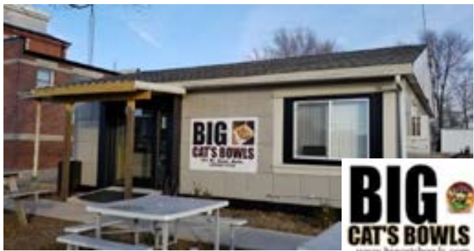
Located at 51 N. 2nd Avenue in Canton
